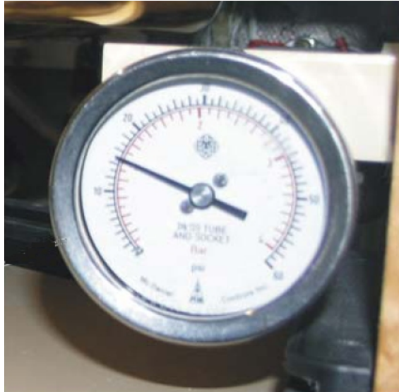
FIGURE 02-38-20-06 - ACCUMULATOR WATER TANK PRESSURE
