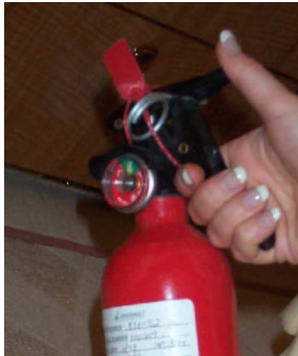
FIGURE 02-25_1-10-01 – EXTINGUISHER SAFETY PIN
