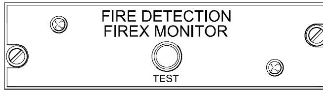
Fire Detection/FIREX Monitor Panel Overhead Panel
