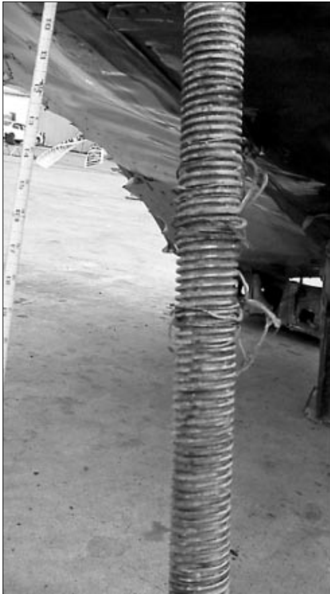
Remnants of thread material sheared from the acme nut can be seen wrapped around this approximately 17-inch (43-centimeter) section of the acme screw. (NTSB photo)
